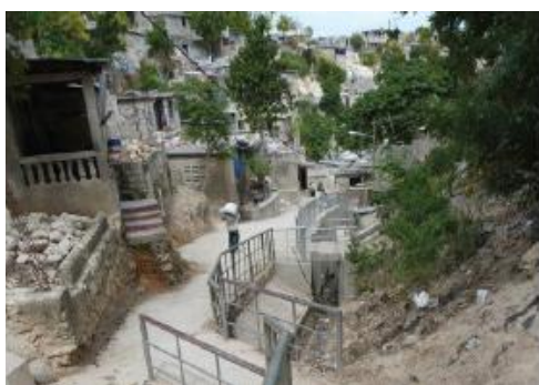
Drainage system upgrade in Martissant 23
