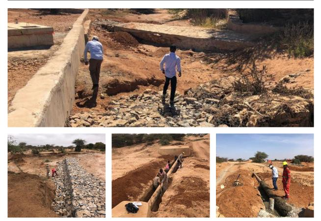
Erosion and flood protection works along critical point of the new pipeline: installation of flood retention walls, gabions, and protection of pipeline sections © UN-Habitat
