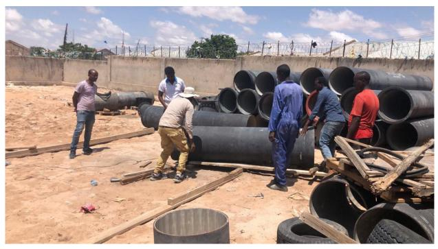
Installation of the final meters connecting the new 23km long transmission pipeline to the Hargeisa Reservoir © UN-Habitat
