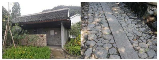
Fig. 3.15 The permeable surface of a walkway to an ecological public restrooms
