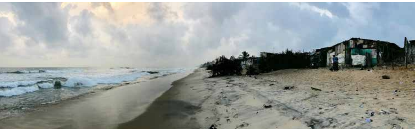
Low standard residential units in Monrovia's coastal area that are susceptible to sea erosion, Feb 2017 © UN-Habitat/Runze Wang
