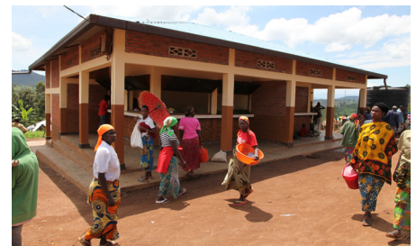
© UN-Habitat Sustainable building for community purposes in Rwanda. Appropriate building design with adequate orientation, sun protection, natural ventilation, use of local materials, and water efficiency technologies like rainwater harvesting. Community buildings can function as showcases and promotion of sustainable building
