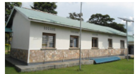
Permanent ventilation in building in Savannah Climate. Uganda. © UN-Habitat / UMU
