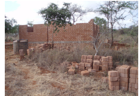
Local building materials: Stone and stabilized soil blocks. © UN-Habitat (top); © Shortie (bottom)
