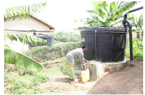
Rainwater harvesting to collect, convey and store rainwater from roofs © UN-Habitat
