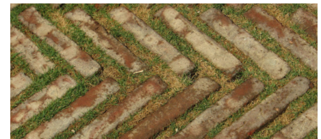
Example of permeable paving to promote water natural infiltration © Ron Mader
