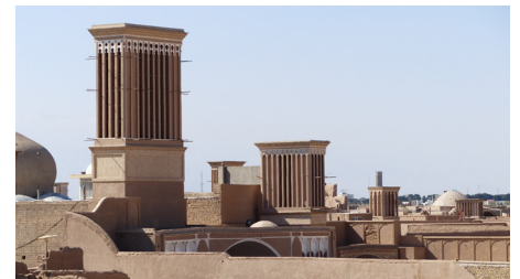
Natural cooling through wind catcher towers © UN-Habitat / Zeltia Gonzalez Blanco
