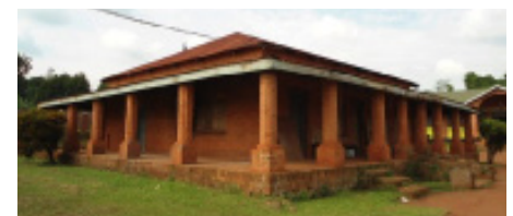
Building protected with solar devices in Lake Region. Uganda © UN-Habitat / UMU
