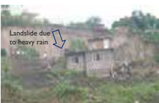
Landslide due to heavy rain Building code alone does not save a building if it is not built on a safe site. If a risky site cannot be avoided, then instead of overinvesting for the sake of building code compliance, constructing a light structure would be wiser. Image: http://fepushahid.blogspot.com/2012_09_16_archive.html
