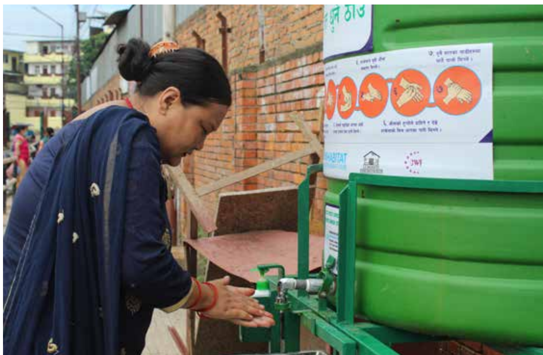
A newly installed touchless handwashing facility by UN-Habitat aims to prevent the spread of COVID-19 in Kalimati Vegetable Market in Kathmandu, Nepal © UN-Habitat Nepal
