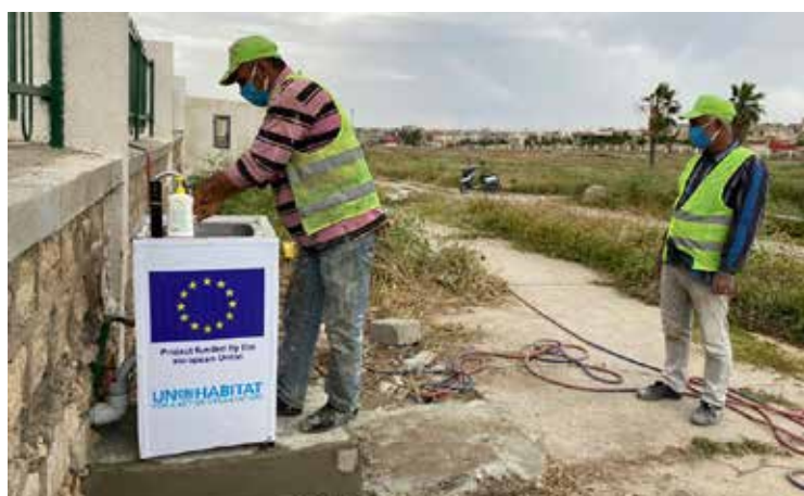
Locally produced handwashing stations installed to prevent COVID-19 spread © UN-Habitat
