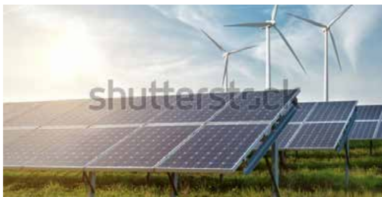
Solar panels and wind generators © Shutterstock
