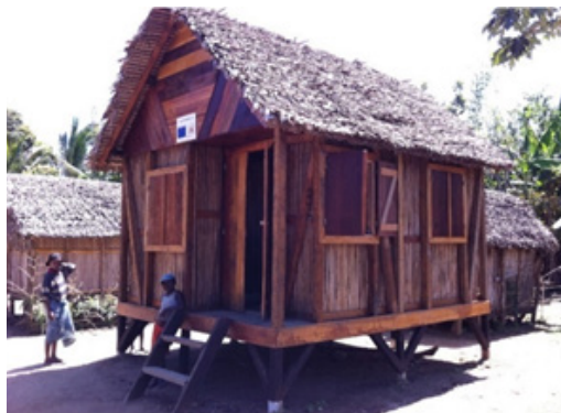
Figure 14: Low-cost anti-cyclonic individual houses using local materials in Maroansetra, Madagascar. Medair, UN-Habitat
