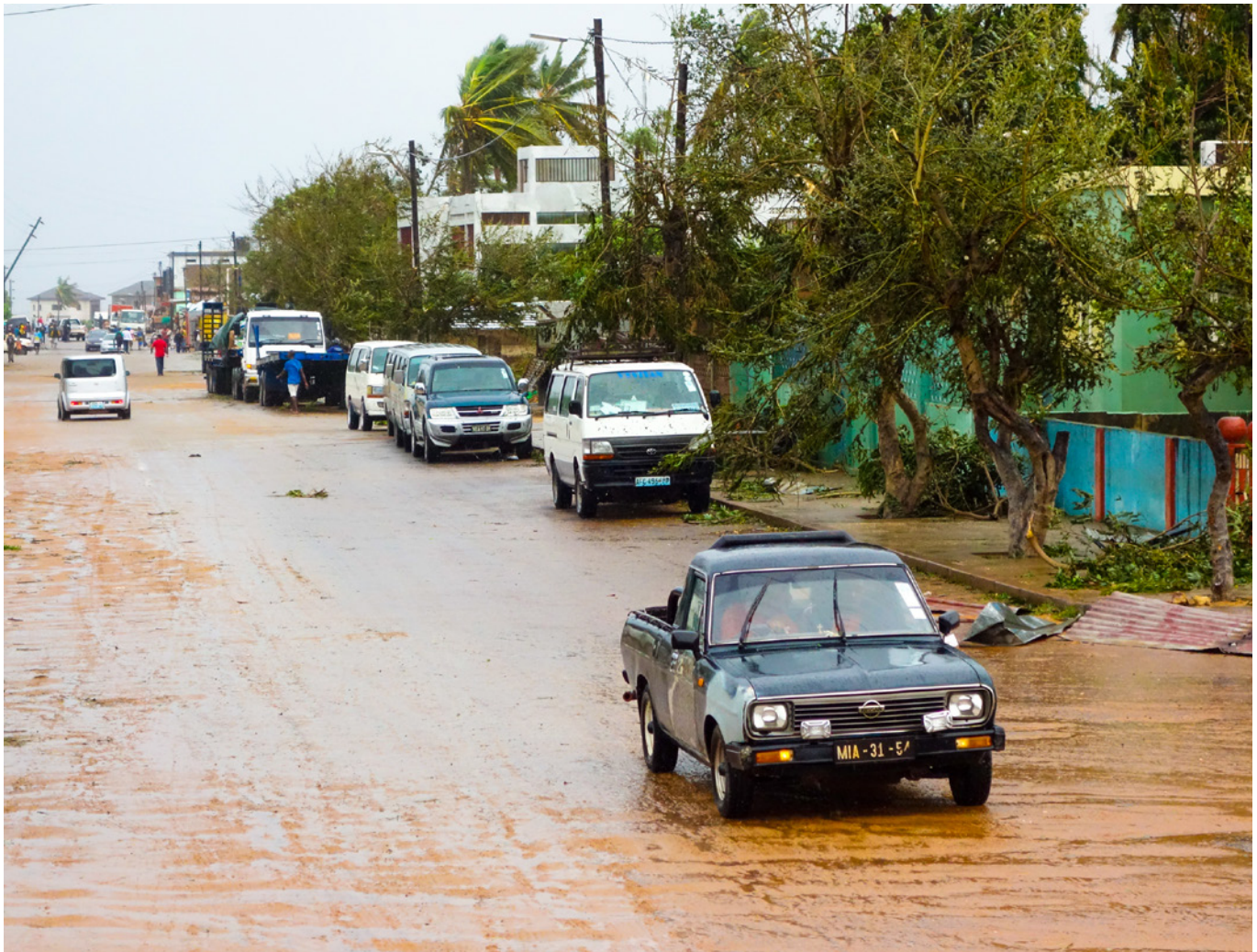
A tropical cyclone destruction at the center of Maxixe city, Mozambique © Shutterstock/Tonis Valing
