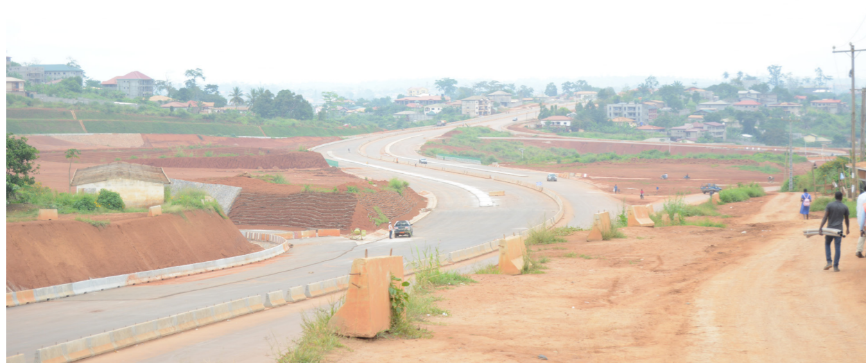
📍 A section of the Yaoundé-Nsimalen highway corridor © UN-Habitat
