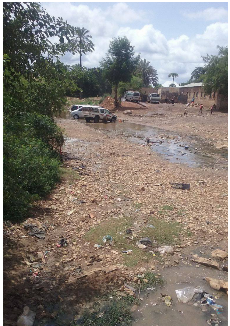
Current condition of the Isha Spring
