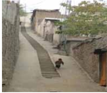
Figure 46: Village road and stairs, renovated in Swat.
