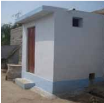
Figure 37: Well-built and maintained latrine in Sindh
