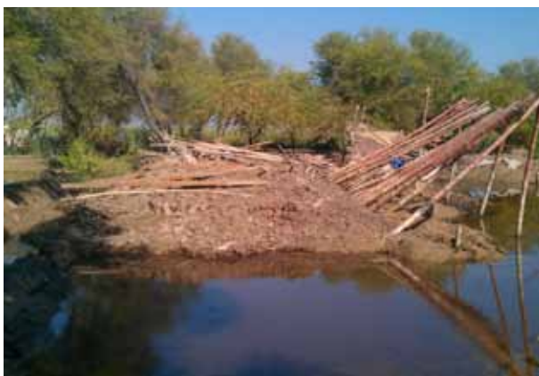
Figure 4: Adobe house dissolved
