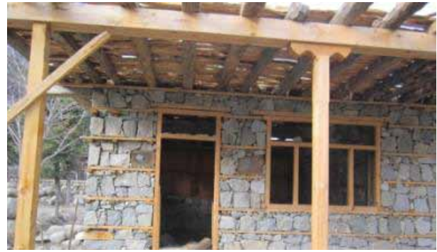
Figure 28: Bhatar house, on-going Construction
