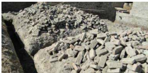
Figure 6: Collapsed house of sun-dried bricks with mud mortar in foreground
