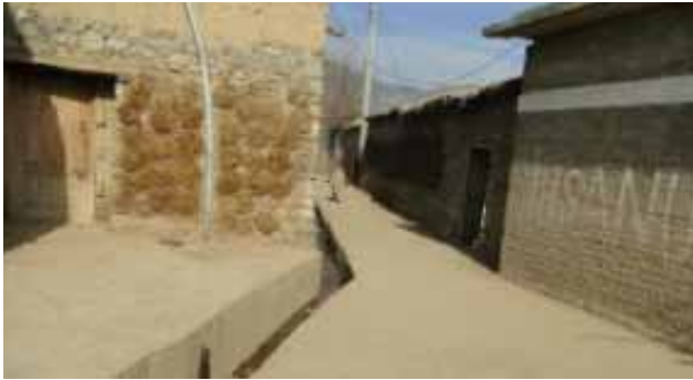
Figure 48: Community-led repair of village interior road in Bajaur Agency
