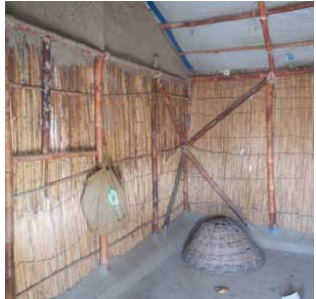
Figure 21: Loh-kat house interior
