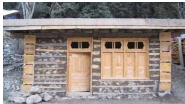
Figure 29: Highly seismic-resistant Bhatar house in Bajaur, FATA
