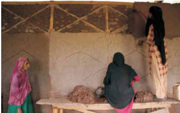
Figure 31: Women plastering exterior
