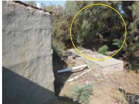
Figure 38: A septic tank connected to a latrine
