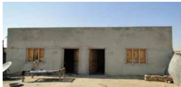
Figure18: Good quality fired-brick shelter
