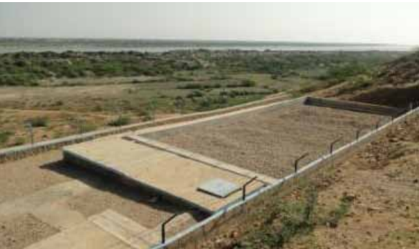
Figure 50. Wetland. The villagers and the CBO had no idea of its utility and how it can be maintained, as there is little water from upstream. According to the UN-Habitat manual on Community Infrastructure, a wetland is used to filter solid human waste and is planted with greenery. However, it is not clear if this PKR5 million project was built by UN-Habitat.
