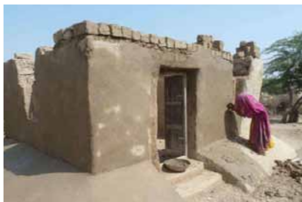
Figure 27: The "toe" foundation
