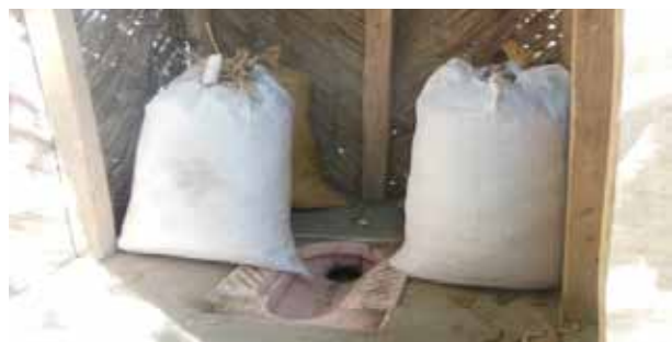
Figure 36: Due to a lack of water, latrines in Sindh wind up as storage rooms.
