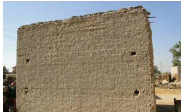
Figure 15: Bitumen and pointing in katcha
