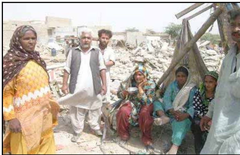
Recent demolitions in Sikander Goth, Pakistan (Photo: URC)
