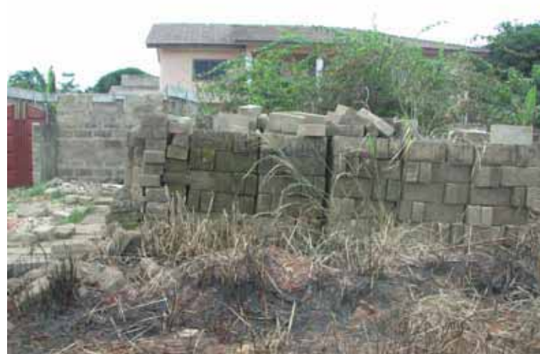
Figure 31. Block saving Photo © G Tipple
