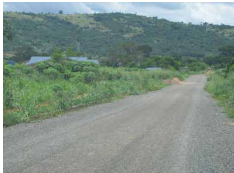
Figure 50. Roads laid ahead of development are under-used for years Photo © G Tiplle
