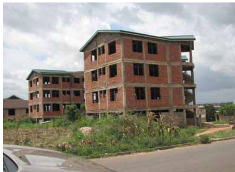
Figure 58. Bricks used as infill in concrete framing Photo © G Tipple
