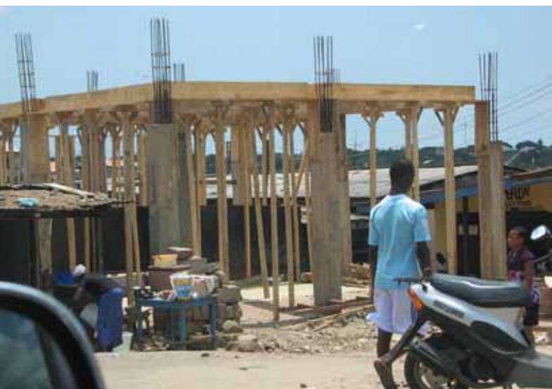
Figure 57. In-situ concrete being cast using wawa formwork Photo © G Tipple
