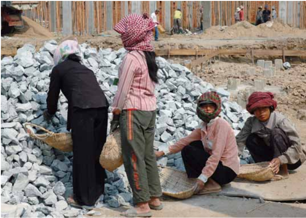
Community members construct their own houses in Borei Keila, Cambodia.
