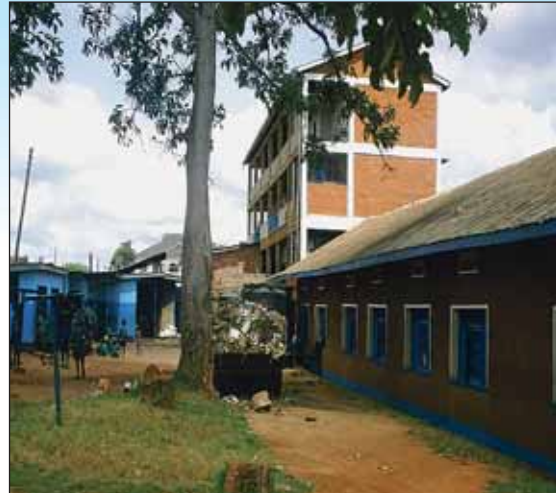
A garbage skip next to the classrooms, Kibuli, Kampala, Uganda.
