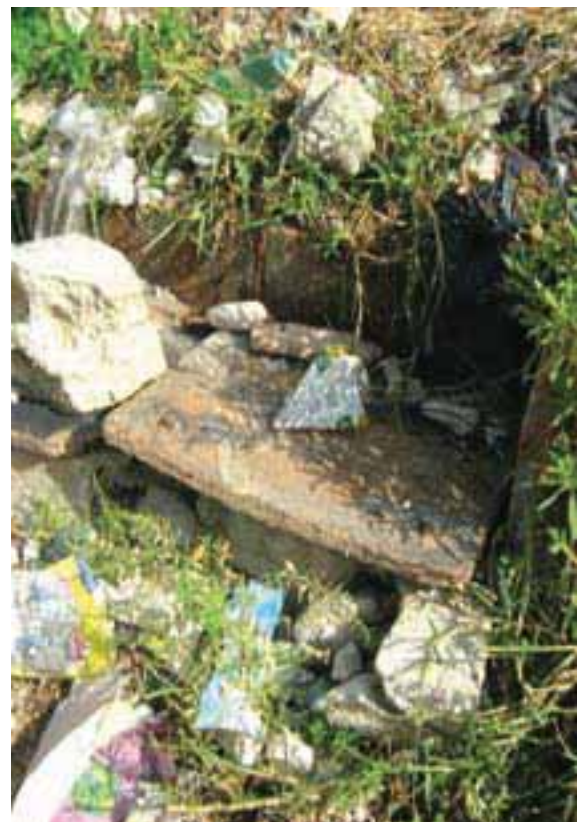
Exposed septic tanks in Jabal el Halib
