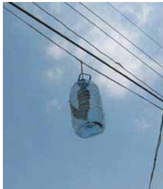
Basic methods for protecting exposed lighting cables in Mouhajarin
