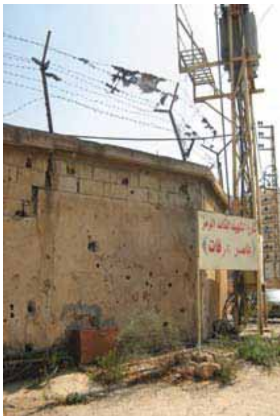
One transformer installed by EDL at the entrance to Tallet el Mankoubin provides electricity to the AA
