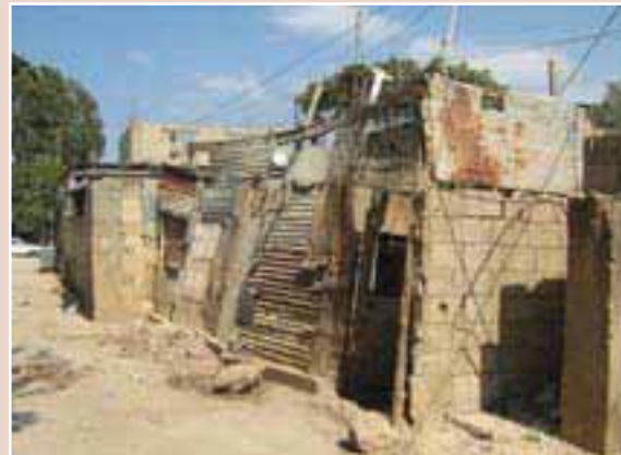
A general view from the AA
