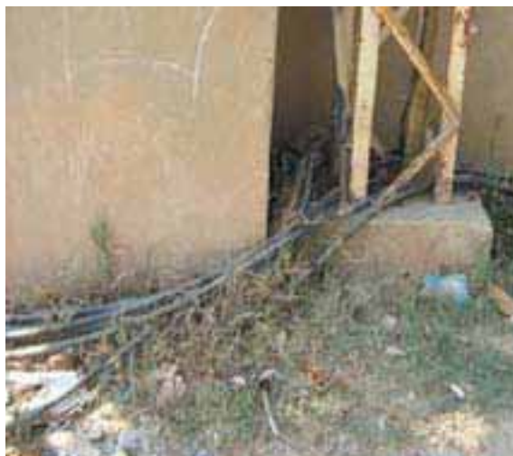
Water reaches houses through above-ground plastic networks installed by dwellers in Tallet el Mankoubin
