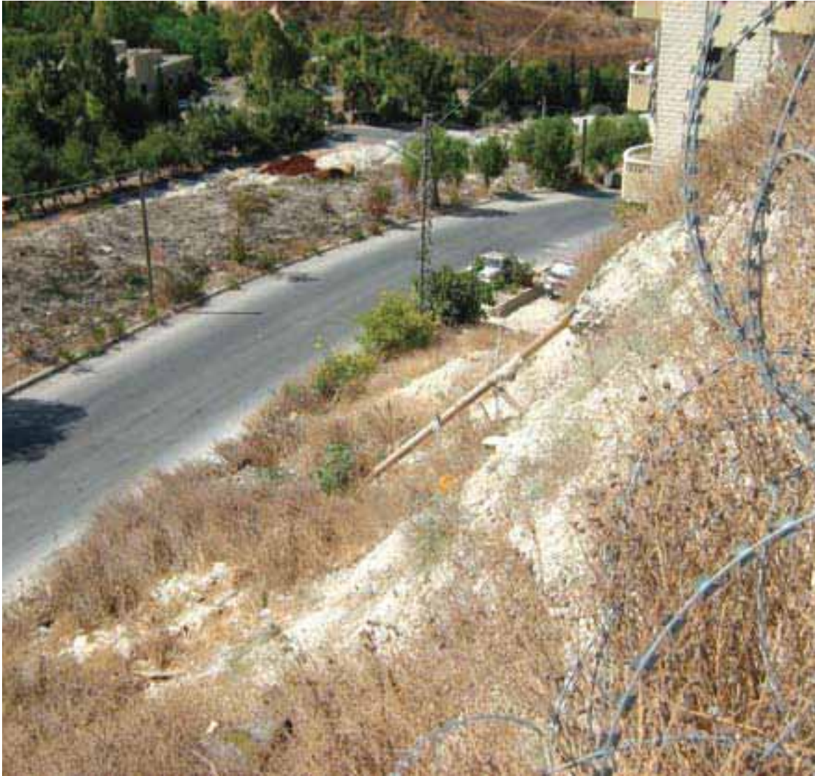
A sewage pipe discharging without proper connection from Hay el Wadi in Mieh Mieh AA to the surrounding Mieh Mieh village in South Lebanon
