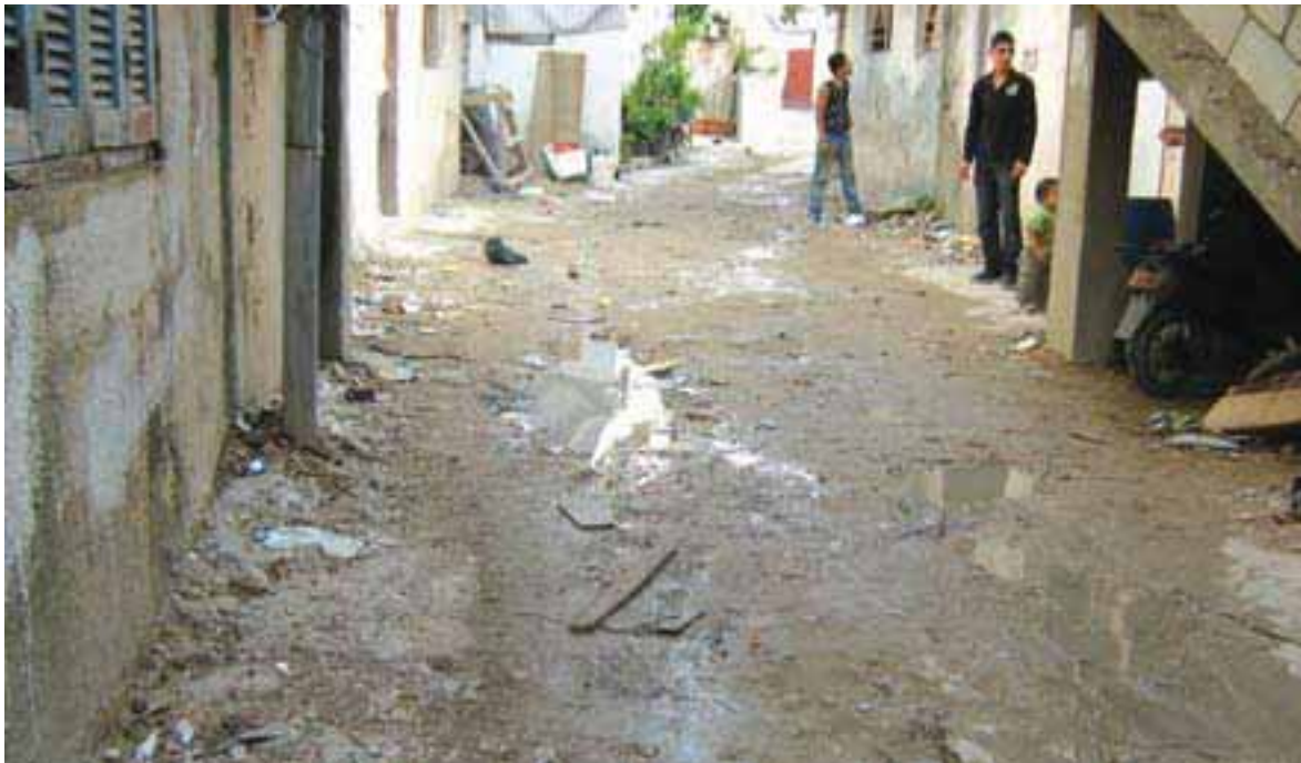
Unpaved internal roads in Baraksat
