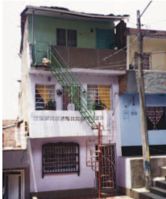
Building rental units require creativity in plot occupation and construction.
