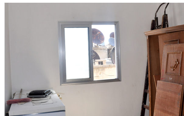
Before and After Photos of shelter rehabilitation in Salah Ad-Deen, Aleppo
