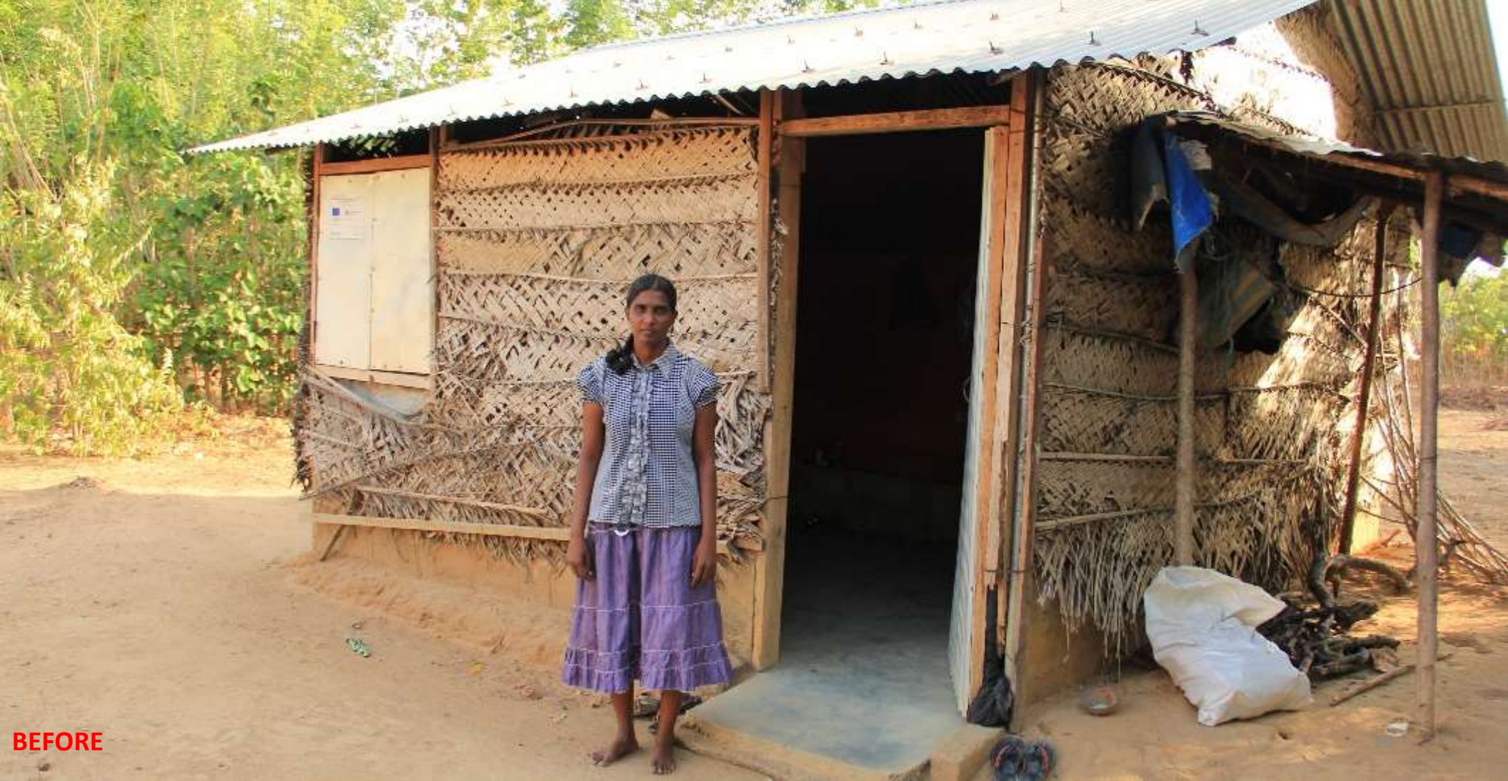
Temporary shelter of a female-headed homeowner in Kilinochchi district, Sri Lanka
