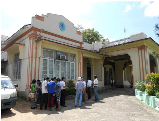
Brick Masonry Building (URML)
