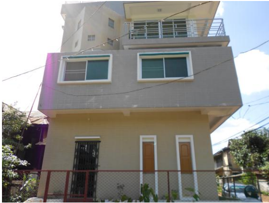
Reinforced Concrete Building (RC)
