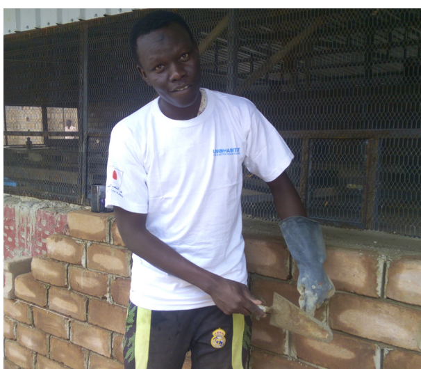
Trained youth engaged in construction work with SSB blocks © UN-Habitat
