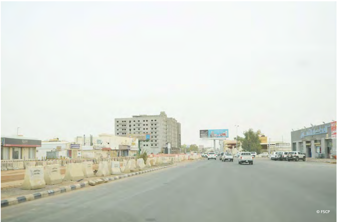
Road infrastructure in Hael
