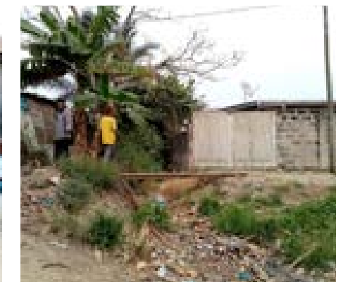
Priority interventions in the neighbourhood of KM4 in Pointe Noire: drainage and accessibility. © UN-Habitat
