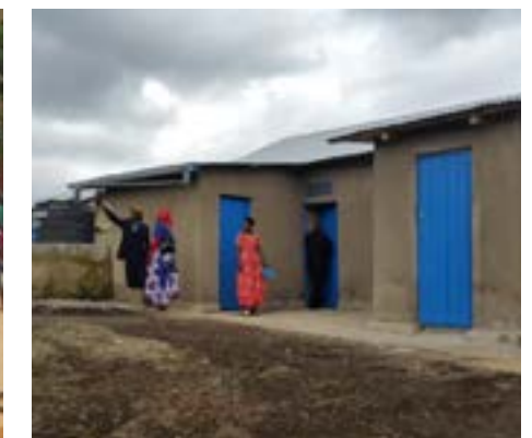
Resilient houses © UN-Habitat Rwanda
