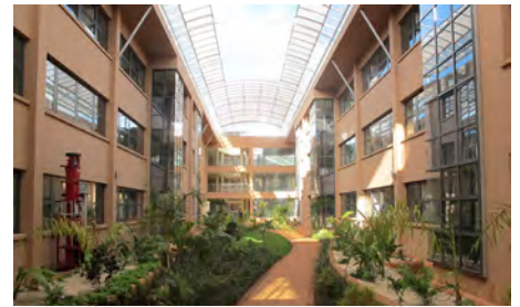
New Office Facility, United Nations Office Nairobi © UN-Habitat / Julius Mwelu
