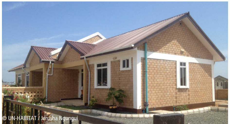
Completed house built with Interlocking Stabilised Soil Blocks
