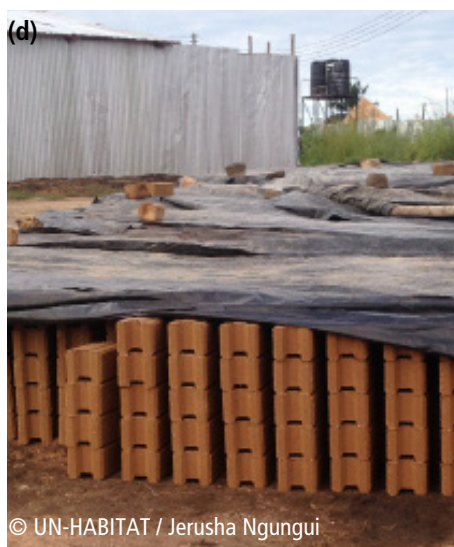
(d) Stacking and curing of the blocks (e) Building using the blocks (f) Resulting block wall
