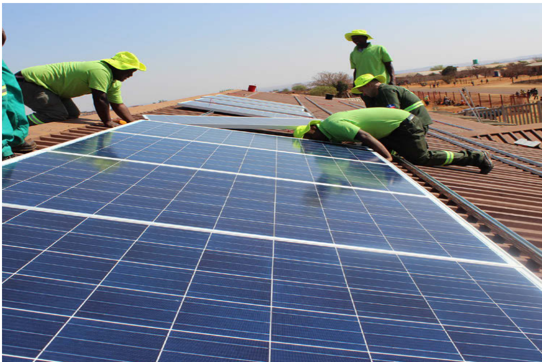
Installation of solar panels in South Africa
