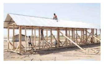
fig.47. Timber structure and iron sheet for Kalobeyei New Site housing
