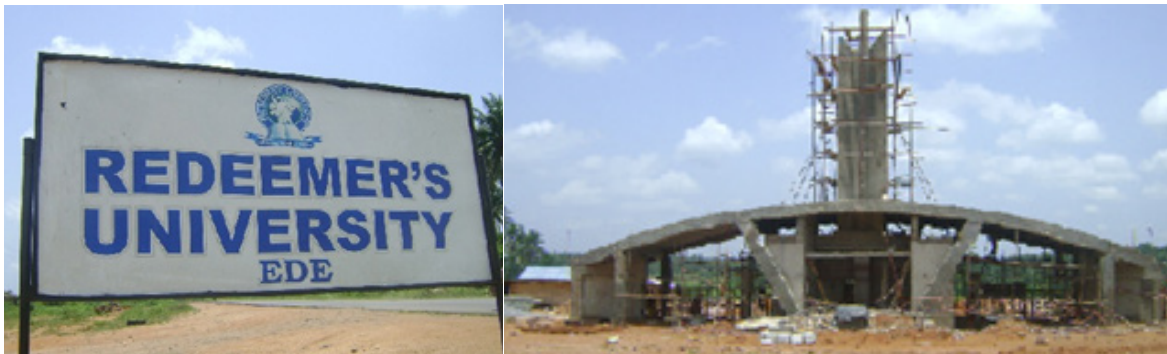
Plate 16: Redeemer's University Ede (under construction)
