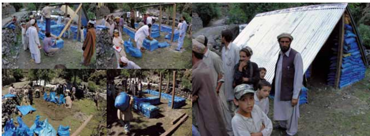
Building one of the transitional shelters Photos: Albert Reichart
