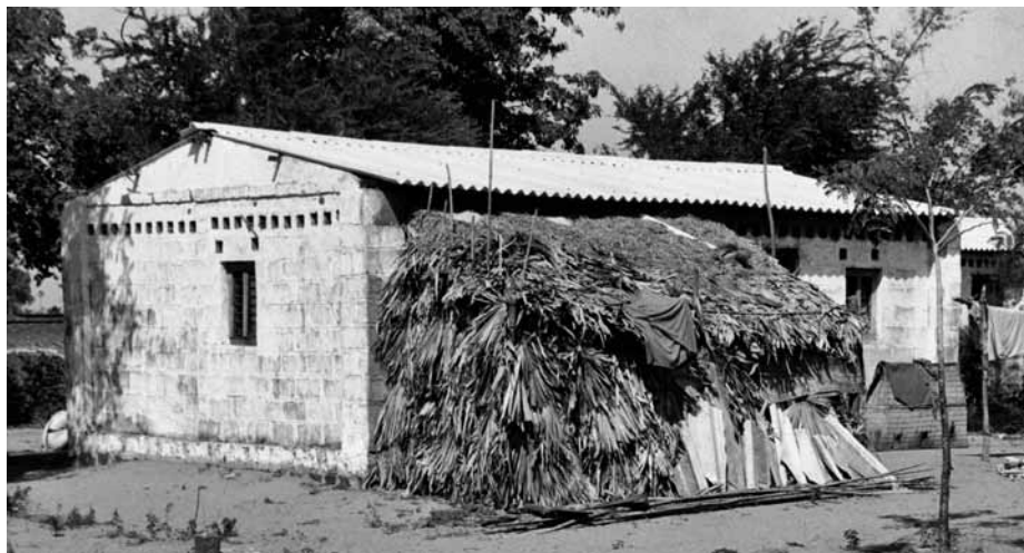
Housing by a reconstruction organisation built in 1969 following the cyclone, with lean to in the foreground. In the village many of the families evacuated most of the concrete block housing to live in improvised thatch lean-tos which are climatically more suitable. Photo: Ian Davis
