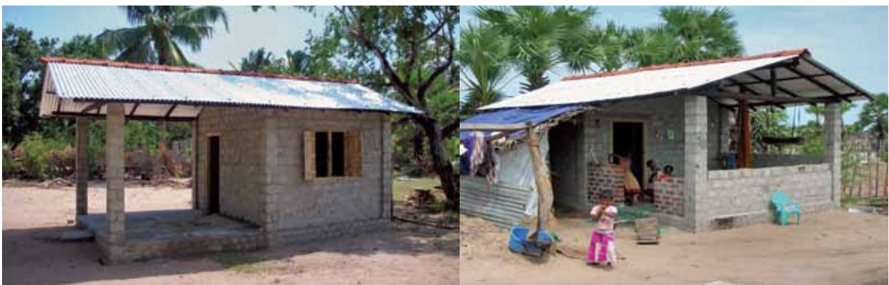
Left: completed shelter. Right: shelter with upgrade by family More than 80% of the families used personal resources or their own time and effort to upgrade their core shelters. Photos: Jake Zarins
