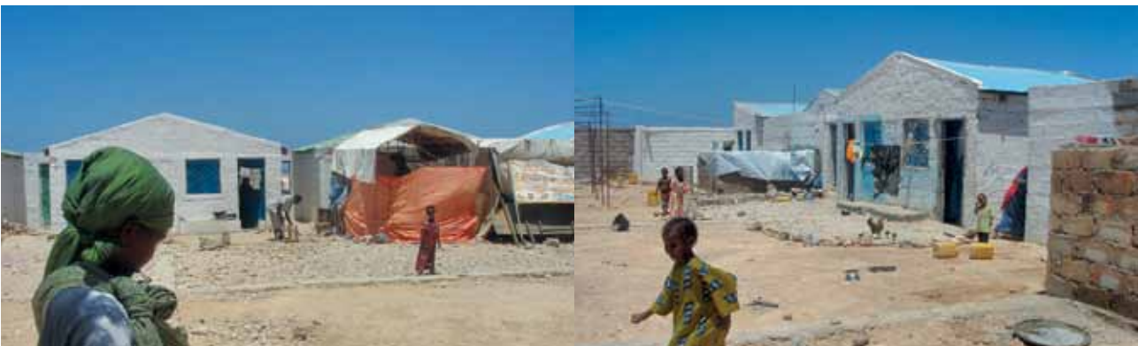
“Sites and services”. The project focused on negotiating land and providing access, secure compound walls, water supply and sanitation for it. Photos: Ombretta Tempra
