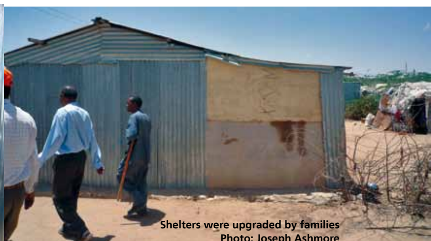
Building a shelter in Hargeisa . Photo: David Womble
