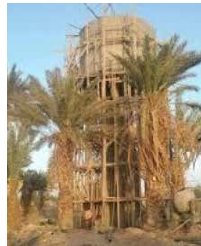
FIGURE 49. Water tower under construction by the Marib
