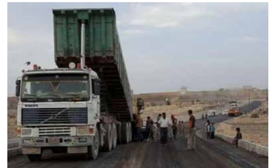
FIGURE 65. Asphaltting in progress (yemen-press.net)
