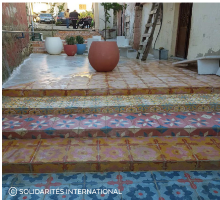
Rehabilitation of stairs and communal spaces of buildings
