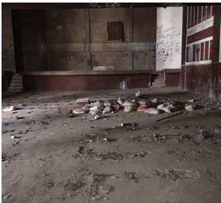
ABJAD Centre before rehabilitation
