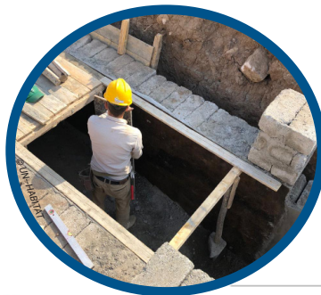
Construction of a culvert box in Sumel
