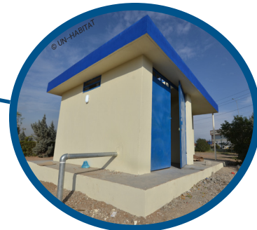
Construction of a new water well in Erbil
