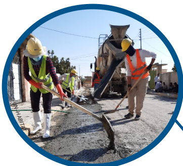
Installation of water pipes in Sinjar
