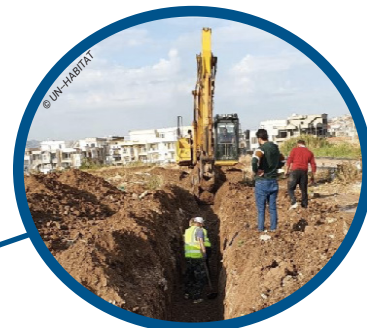
Installation of water pipes in Duhok
