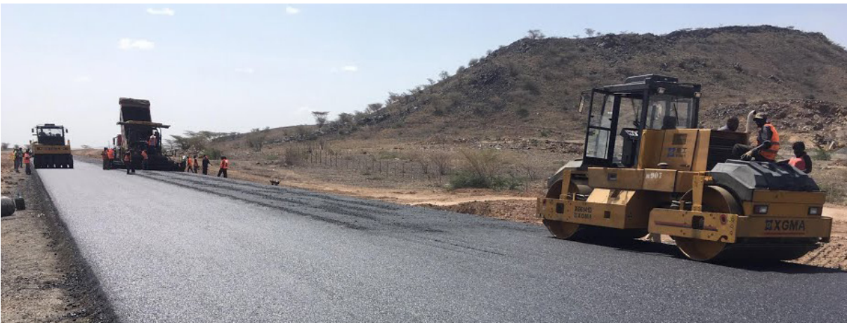
Ongoing construction of Loichangamatak - Lodwar - Nadapal/Nnakodok highway. © KENHA.
