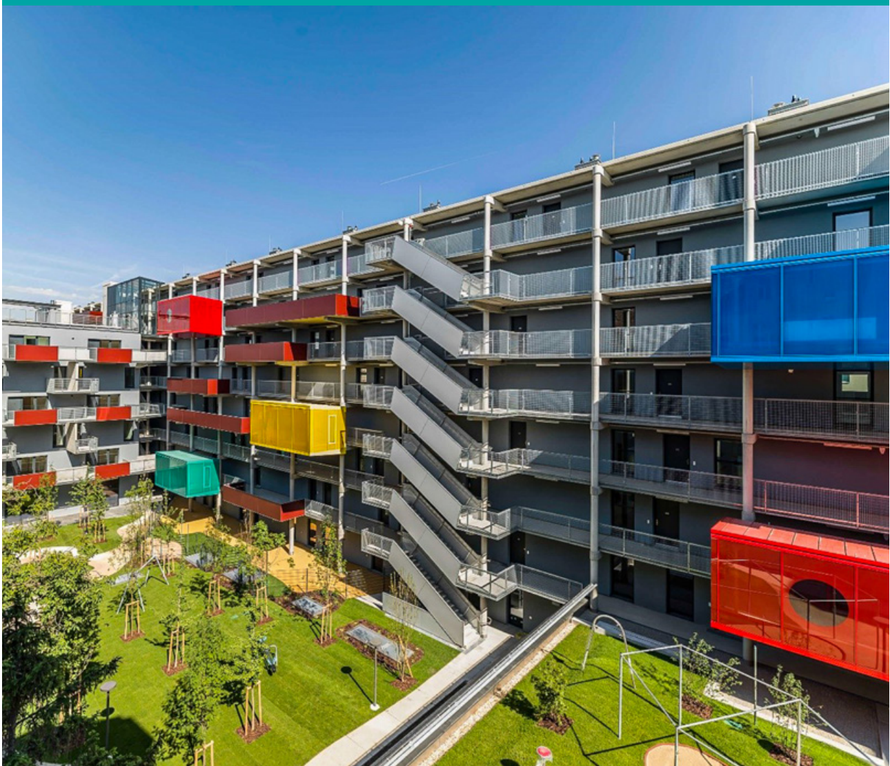
Photo 3 Social housing development in Vienna, Austria
