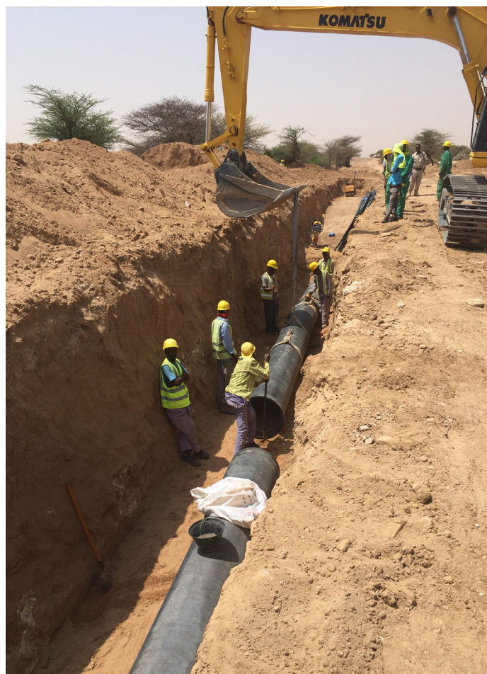
A section of the 23KM pipeline
