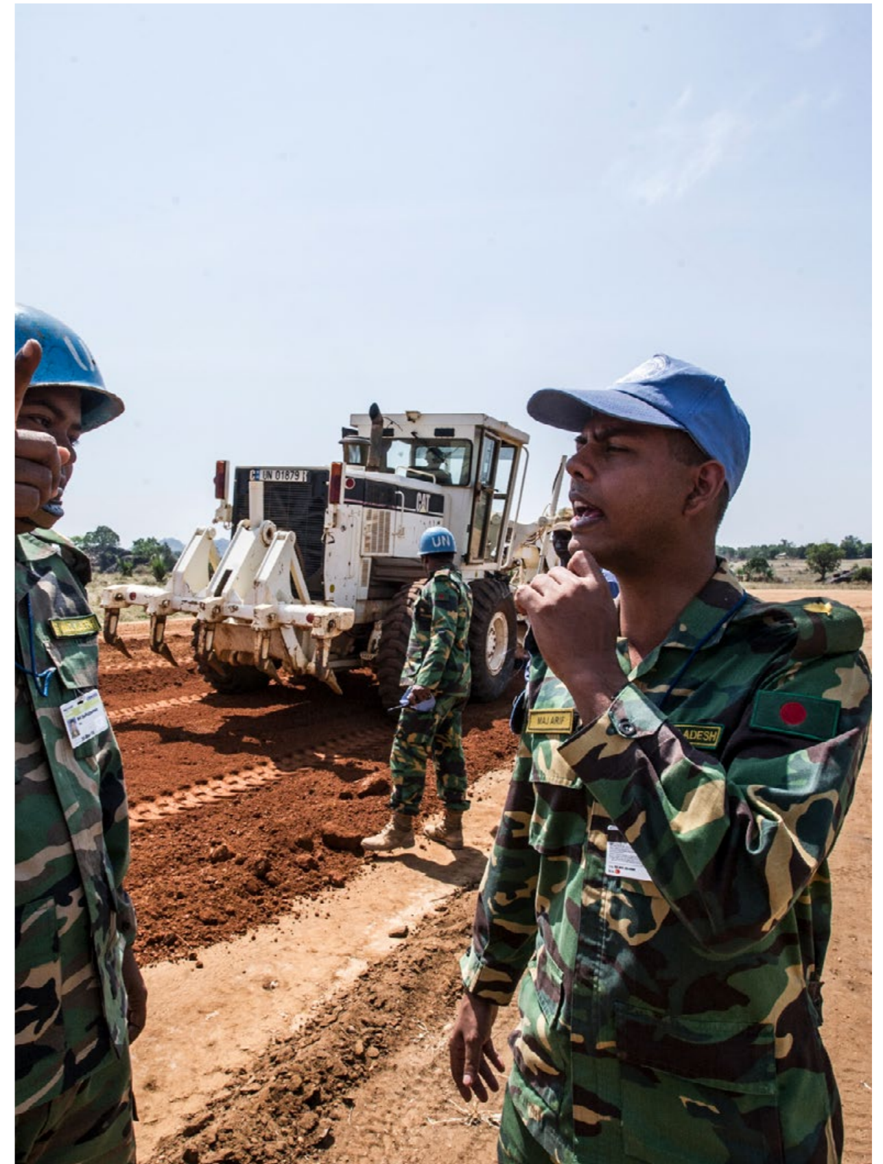
Figure 8: Mangalia road construction by UNMISS. ©United Nations, (UNMISS), 2014
