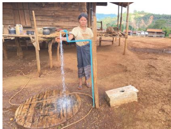
WASH System placed in Sekong, Lao PDR © UN-Habitat
