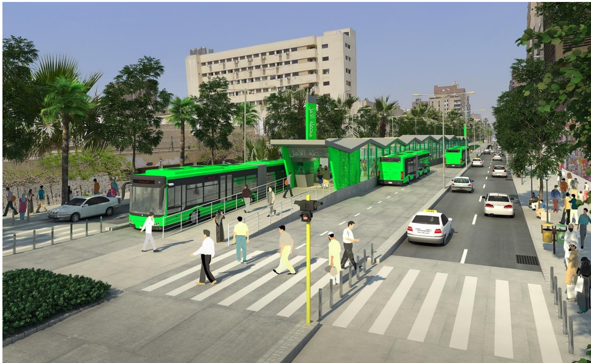
Figure 7. The BRT will incorporate high-capacity buses, centrally aligned stations, passing lanes, and safe pedestrian access.
