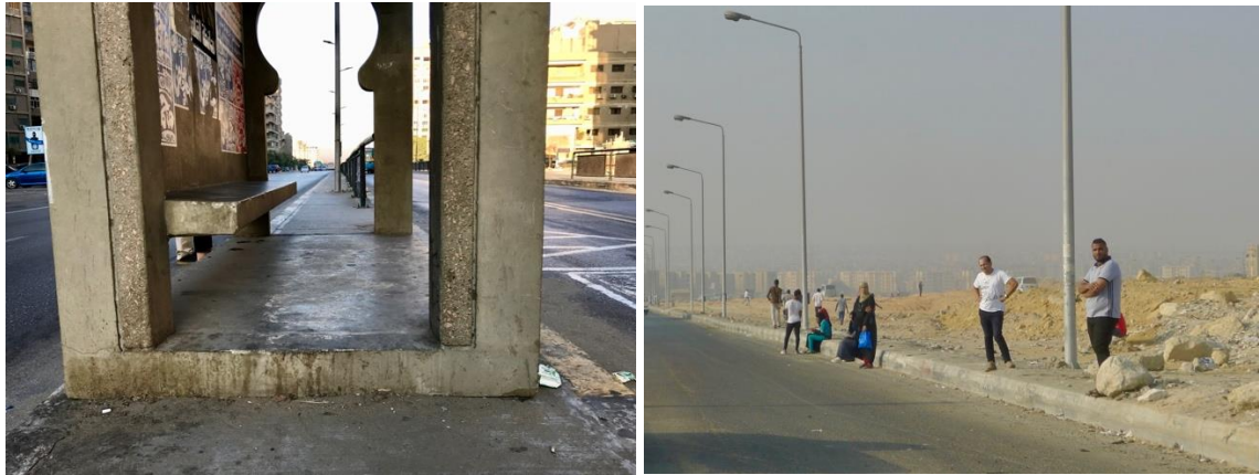
Figure 28: Bus shelters recently installed in Cairo have a large step, thereby compromising access for persons with disabilities. In the new communities, shelters are often absent.
