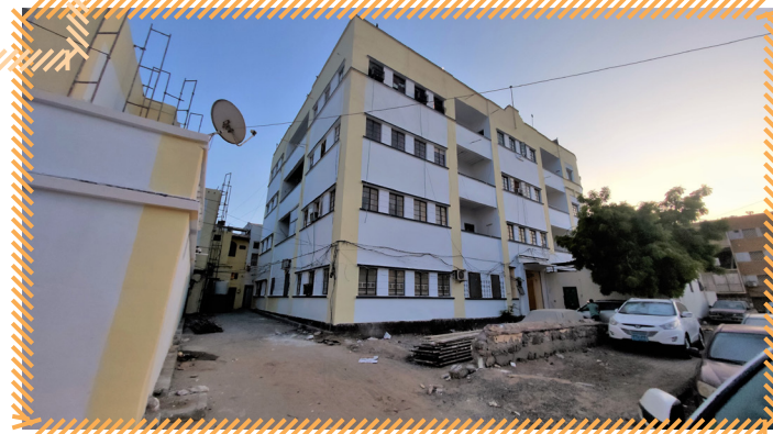
A building before and after rehabilitation under “Adequate Housing” project, Yemen. Photograph: UN-Habitat
