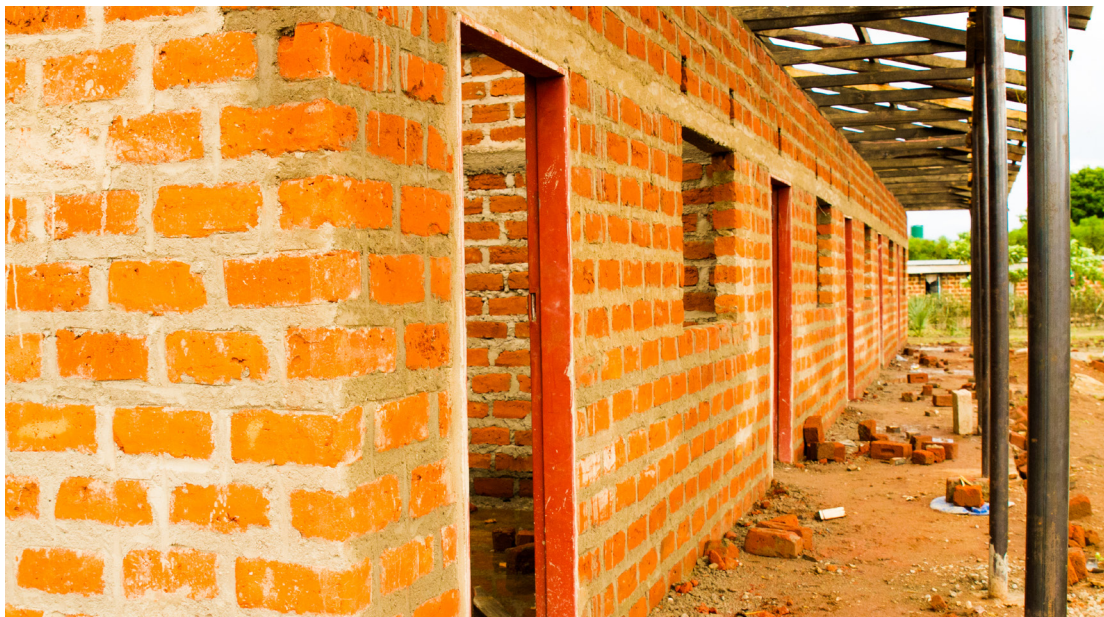
Red pan brick building for a classroom and toilet construction. © Shutterstock/ FANKS
