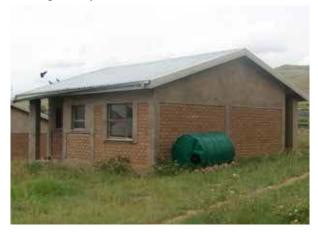
FIGURE 84 Hydraform blocks are laid without mortar
