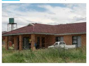
FIGURE 60 Water tank for roof run-off
