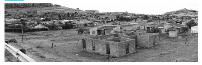
FIGURE 73 Informal construction using high quality materials; machine cut stone and local bricks
