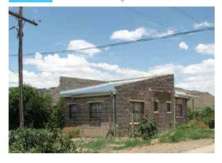
FIGURE 82 Cement block housing by MLGCPA
