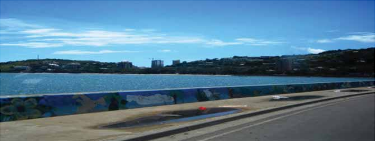
Koki to Ela Beach Seawall Photo © Auka, J., 2013
