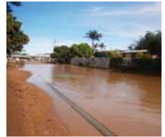
Poor drainage system resulting in overflow of water onto the road at the Rainbow residential area. Photo © Miria, G., 2012
