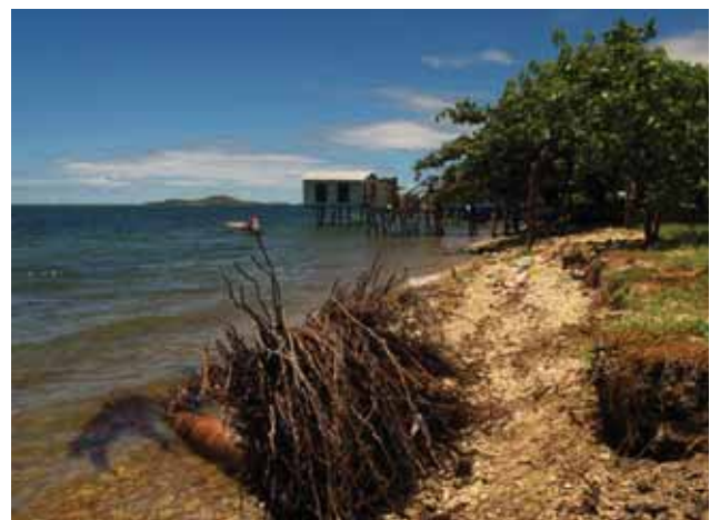
Accelerated coastal erosion - the two pictures were taken less than six weeks apart Photo © Miria, G., 2012
