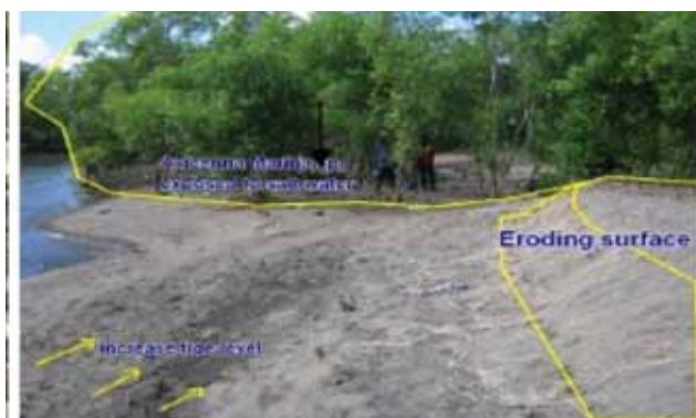
Coastal Erosion in Port Moresby Photo © Kaluwin, C., 2008
