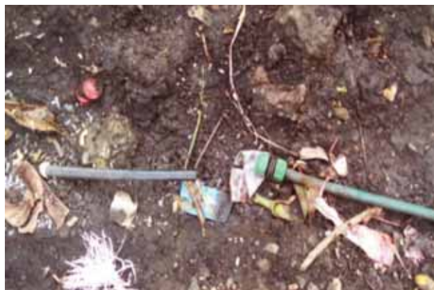
(Left) Illegal water usage (Right) Vandalized water pipe Photo © Susuki, W. and Newalli, J.
