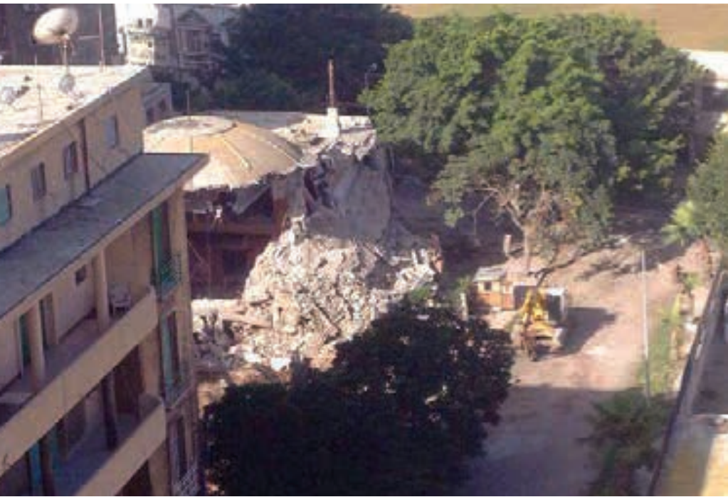
Demolition of Villa Aghion, Alexandria
