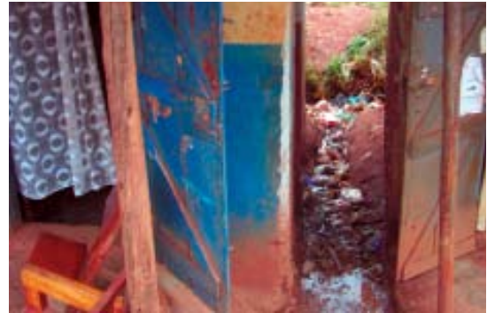
Poor drainage. Photo: © Kampala city council
