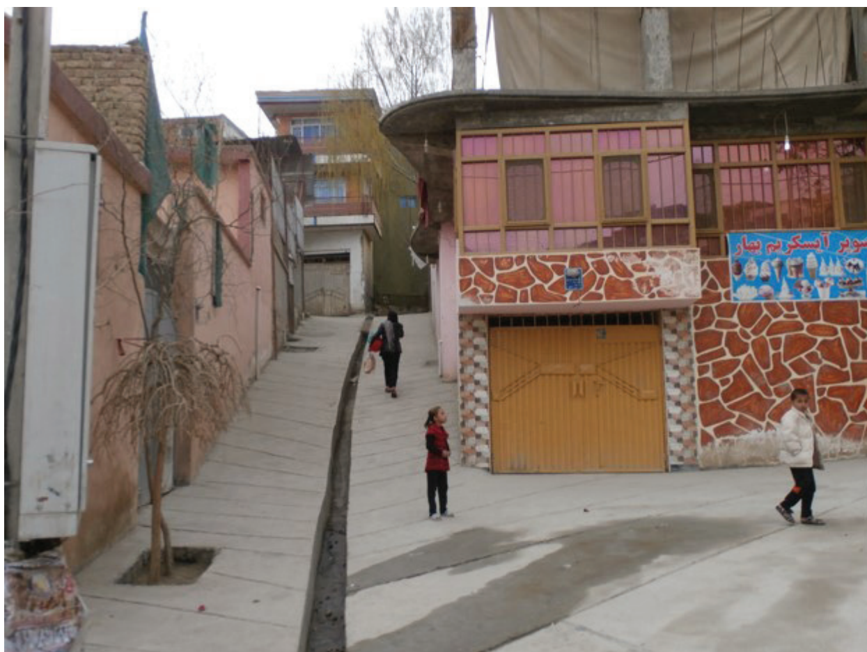
FIGURE 42 IMPROVED ROAD DRAINAGE HAS SHOWN TO LEAD TO HOME IMPROVEMENTS
