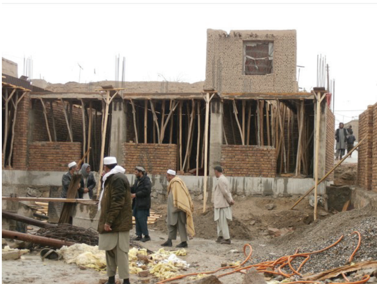
FIGURE 52 A SINGLE-STOREY BUILDING UNDER CONSTRUCTION
