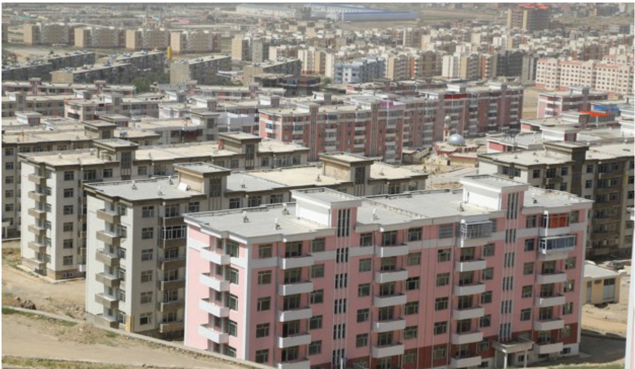
FIGURE 26 THE 2,104 UNIT KHWAJAH RAWASH HOUSING PROJECT
