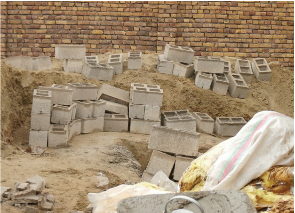
FIGURE 50 HOLLOW CONCRETE BLOCKS ARE LOCALLY MANUFACTURED, THOUGH CEMENT IS EXCLUSIVELY IMPORTED
