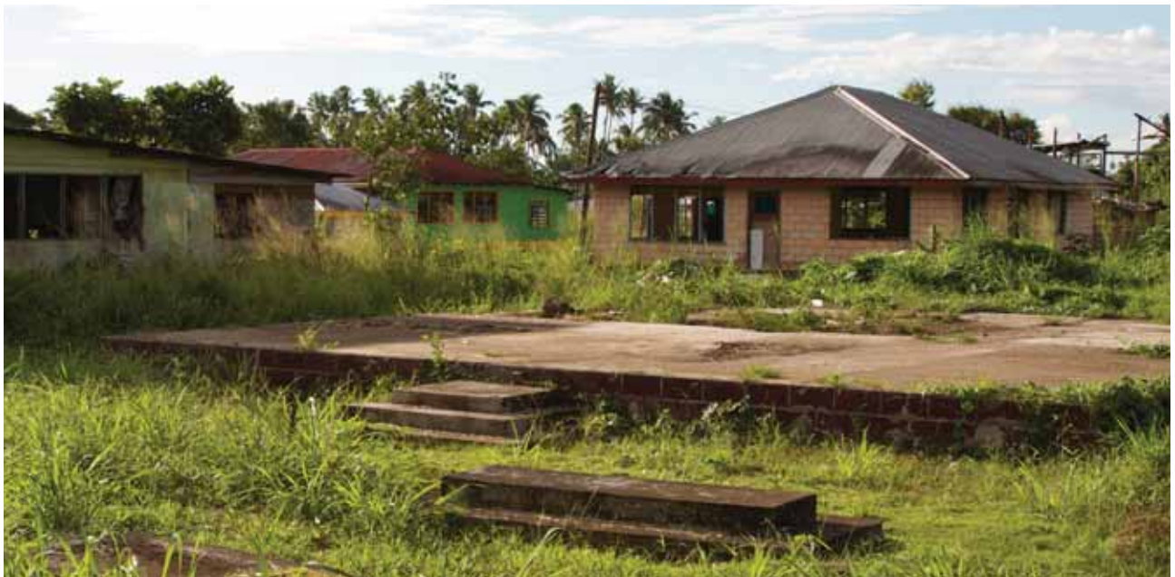
Damaged housing in Apia, post- Cyclone Evan, 2012 Photo © UN-Habitat / Bernhard Barth
