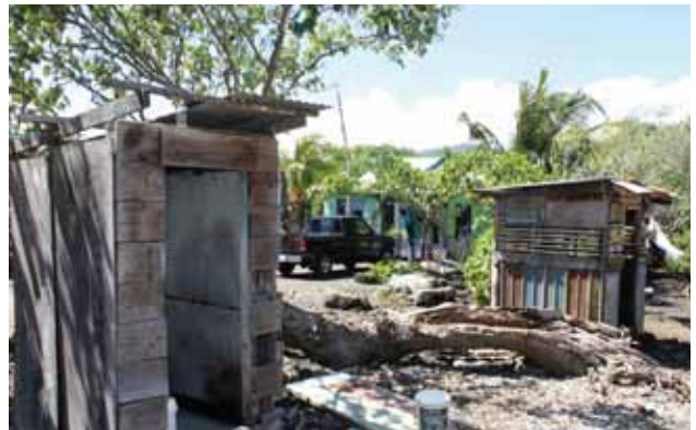
Sanitation systems in a vulnerable village in Apia. Photo © PUMA, MNRE, Samoa
