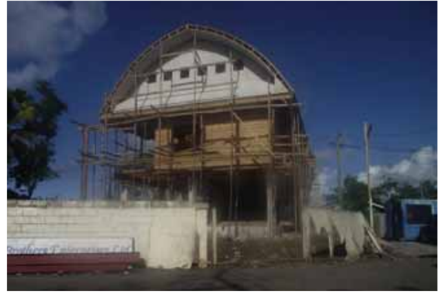
Concrete fences and elevated floor levels for flood protection.
