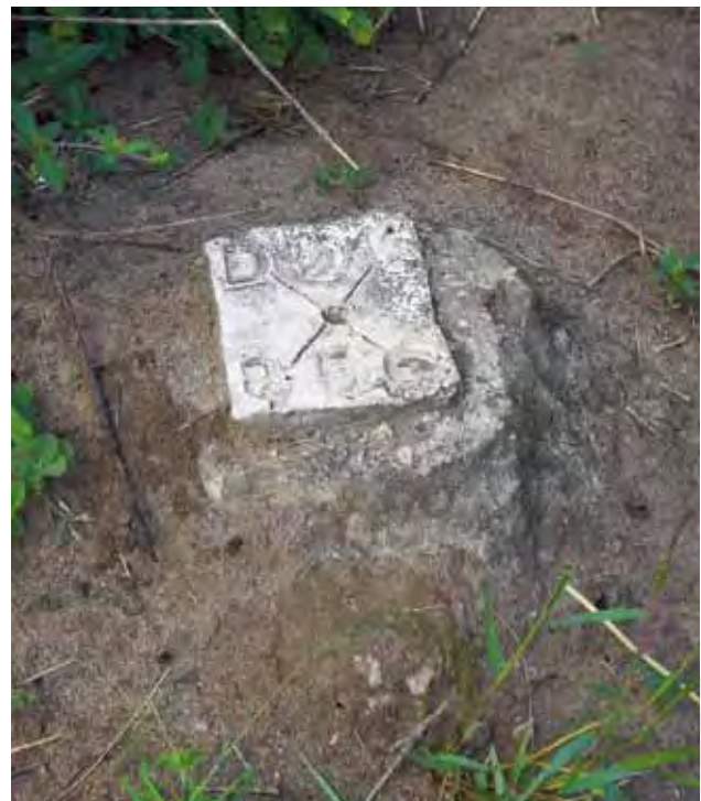
Plot beacon in a planned new land development scheme Photo © Rasmus Precht
