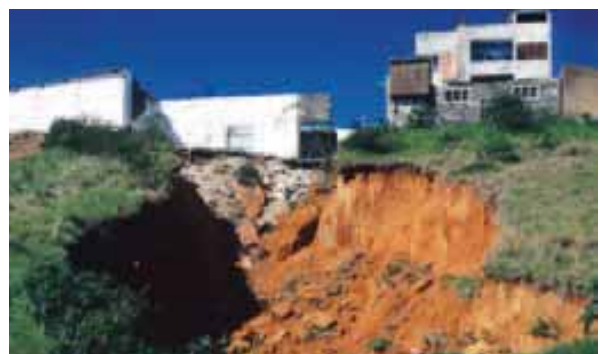
Soil erosion, Maputo © UN-Habitat/Jesper Milner
