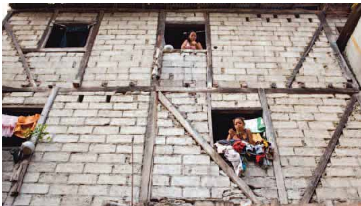
Composite construction, cement and wood are a relatively inexpensive solution to the problems of self-owned houses in Esmeraldas, Ecuador
