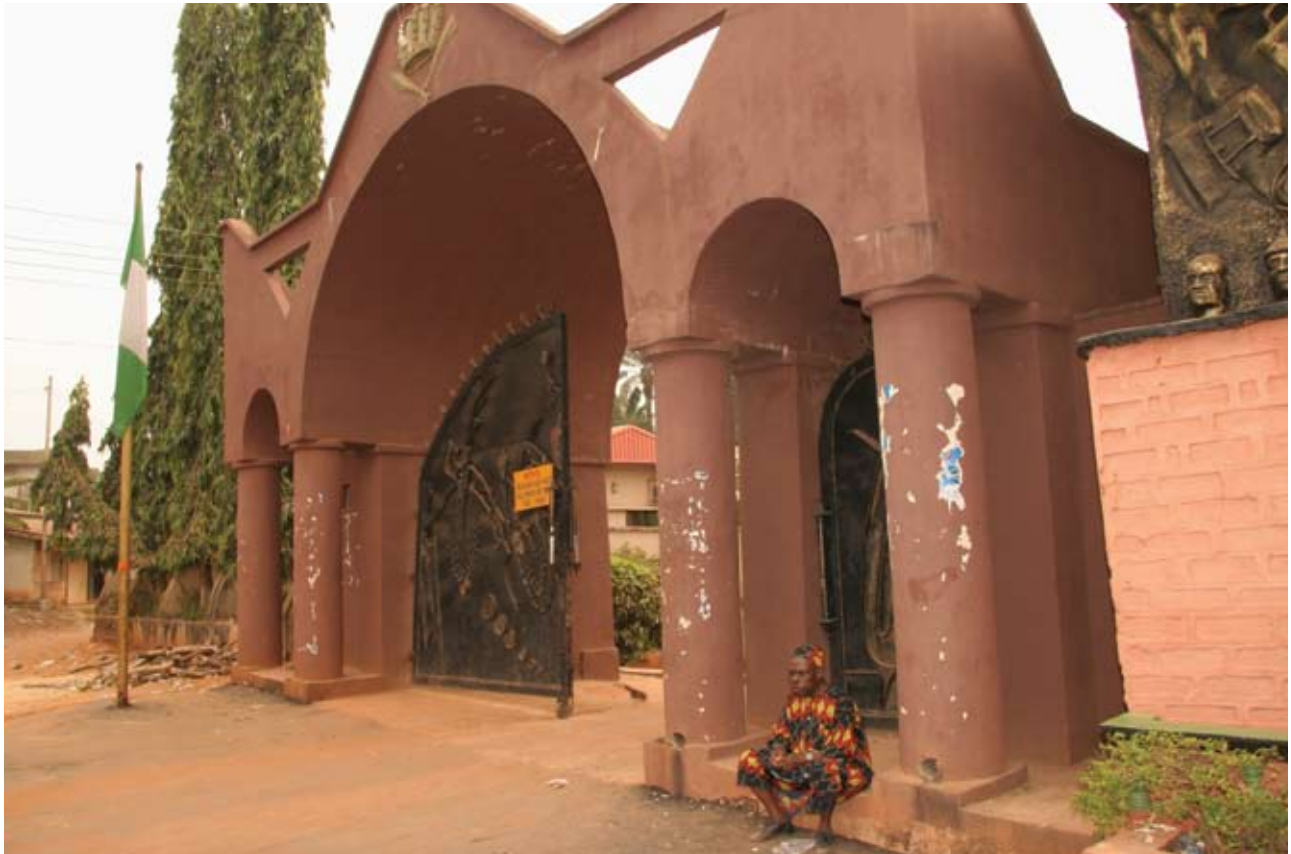
FIG 3.19: VIEW OF THE IMPOSING ENTRANCE OF THE OBI'S PALACE AT AWKA.
