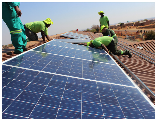
Solar Panel installation in South Africa Urban-LEDS © Grace Stead
